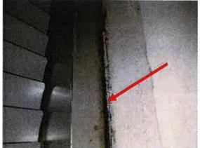
Photo #18 Black/white caulk ("H") on the perimeter doors and windows, front office area – contains asbestos
