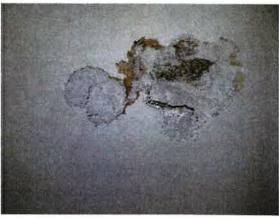
Photo #16 Gypsum wall board ("E") in front area – associated joint compound contains asbestos
