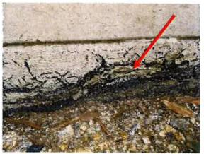
Photo #24 Exterior waterproofing ("Y") on the perimeter concrete foundations
