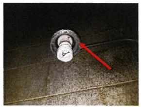
Photo #30 Light fixture gasket ("AF") in the front area HVAC closet – assumed to contain asbestos
