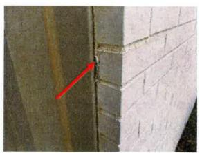
Photo #23 Exterior caulking ("X") on expansion joints, doors, and windows
