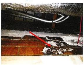
Photo #21 Residual brown mastic ("T") on the brick walls in the elevated work room
