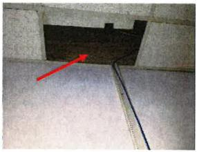
Photo #19 Fireproofing ("J") on the perimeter structural steel ledger, front office area
